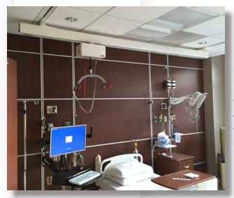
Rail styles include both exposed and recessed. Any room covering system requires that the traversing rail be completely exposed, but the guide rails on a room covering system can be recessed. Straight rail systems can be completely recessed when room design features permit. Recessed rail is more expensive to install but adds a clean look to the room.
