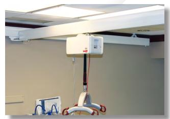
A room covering ceiling track system allows the hoist motor to travel to all 4 corners of the "H" shaped rail system. This design allows for ease of transfer within any point of the room. Lifting is easy on the patient when the hoist can self-center over the patient while coming under load. Available up to 20 ft (6 m) wide by any length.
